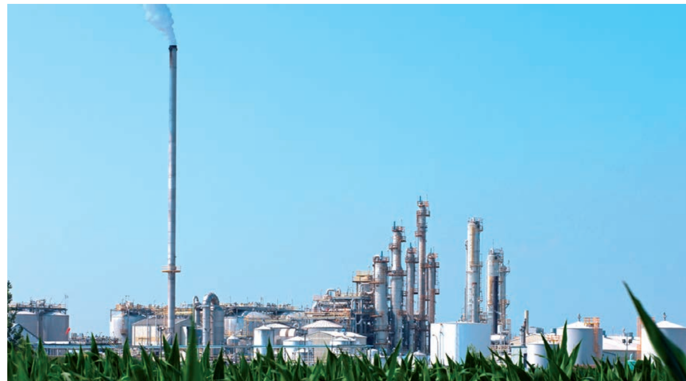
Pyroalliance makes equipment for petrochemical plants.
